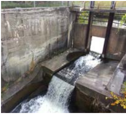
Alcott Street Dam Structure. Credit: USFWS
